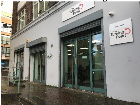
The Designworks building entrance located on Park Parade
